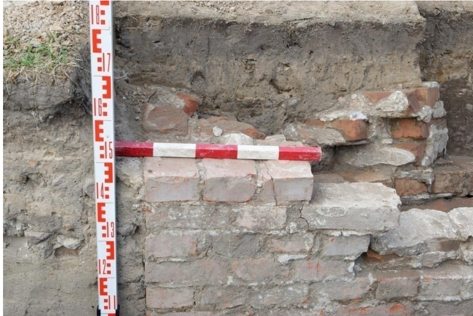
Fig. 68. Main trench, part 4, close-up of a fragment of the northern profile – brick wall ceiling (object 3). Photograph by P. Wlizo
